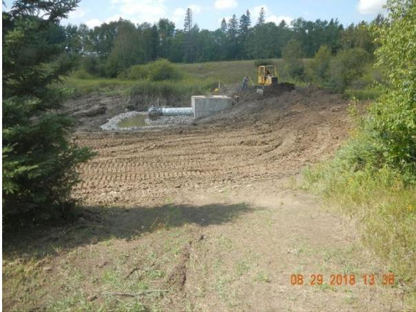
Inlet end of new control structure. Dozer if finishing the embankment for seeding.
